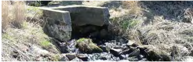
Failing fish passages prevent fish from migrating past man-made barriers to their fresh water spawning sites.
