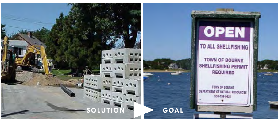
Dry wells and sand filters protect shellfish beds from polluted stormwater runoff.
